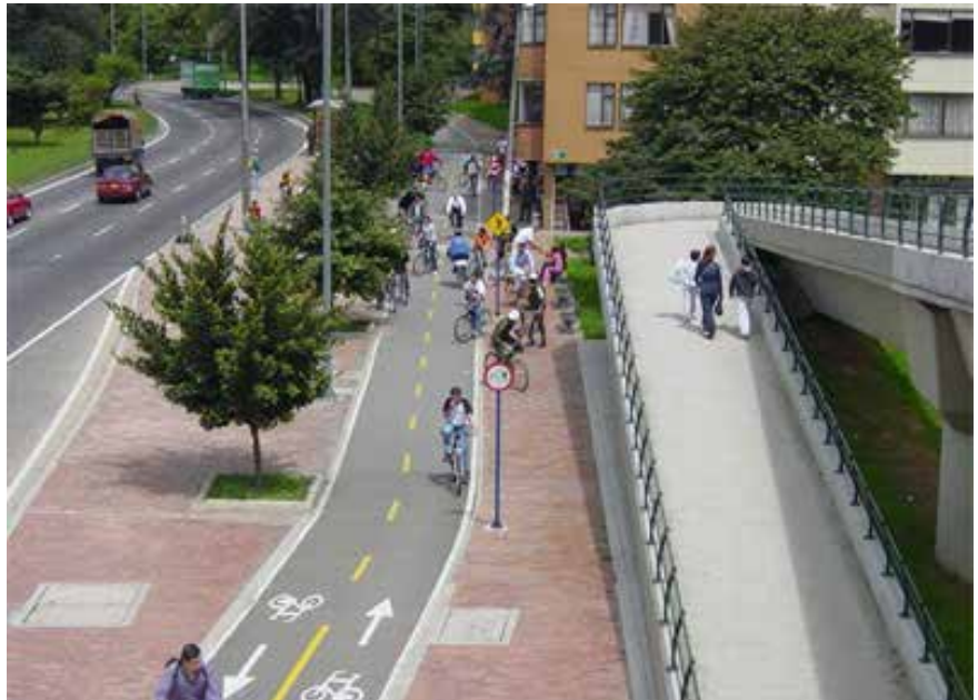
Image 2 - Cycle track separated from main road with wide sidewalks and tree buffer.
