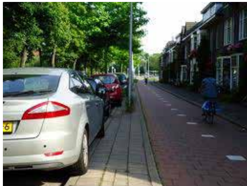
Image 3 - Brick paved cycle track located behind parked vehicles.
