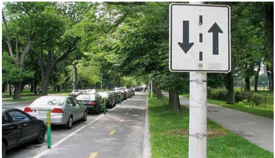
Image 6 - Cycle track located behind parked cars and separated by bollards.
