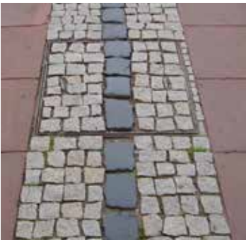
Image 2 - Stone mosaic with a permeable fill between the stones.
