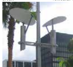
Image 10 - Contemporary fully shielded light fixture bracket mounted at 14' height on a 20' pole - a good method for integrating pedestrian scale lighting with required roadway lighting.
