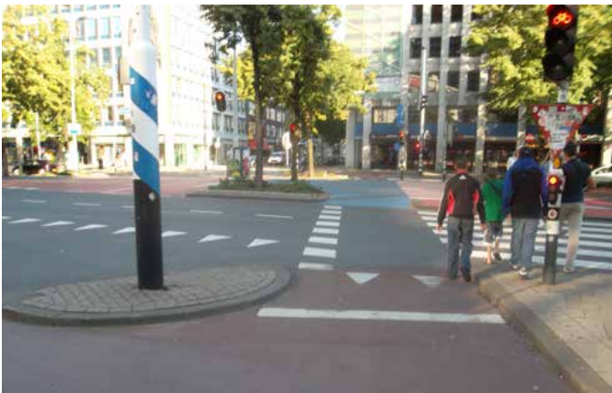
Image 5 - Bike lane at intersection separated from pedestrians
