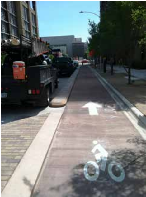
Image 1 - Cycle track separated with concrete and paving.
