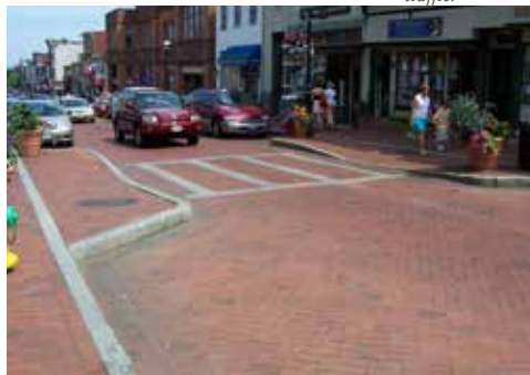
Image 7 - Mid block crosswalk with granite used for curb material.
