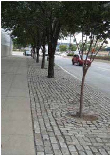
Street tree planted in permeable material
