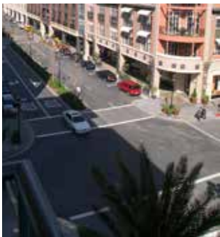
Image 6 - Bulb-out intersection with a clearly defined crosswalk.
