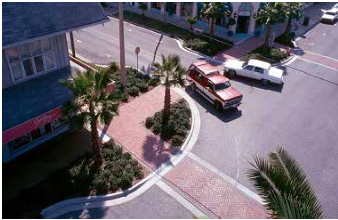
Image 2 - Landscaping integrated into the bulb-out. Notice that there is still a clearly defined visibility of pedestrians allowed.
