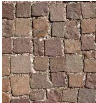
Image 3 - Bricks with sand support a permeable material system.
